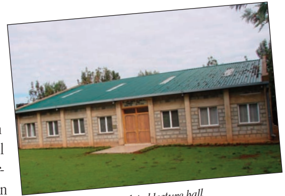
Completed lecture hall
